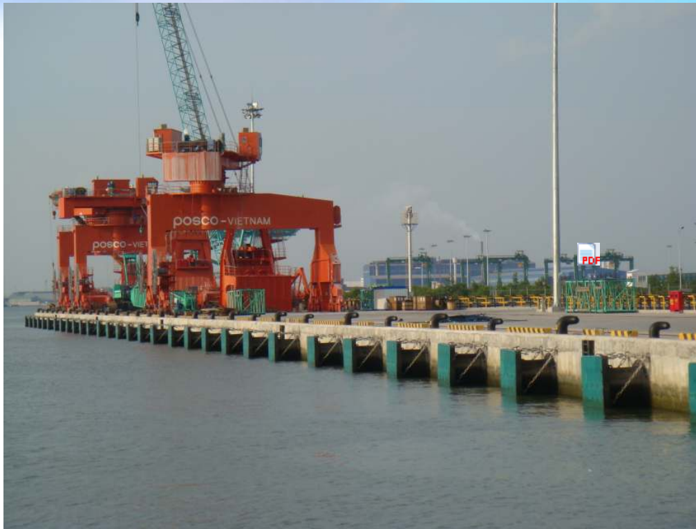
SPOOL FENDER 1450H 32 SETS (PANEL 2200W X 4000L X 250H)
