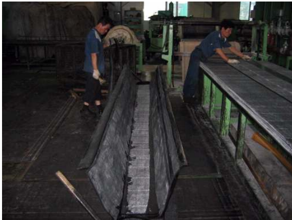
3. MOLDING WORK FOR ARCH FENDER
